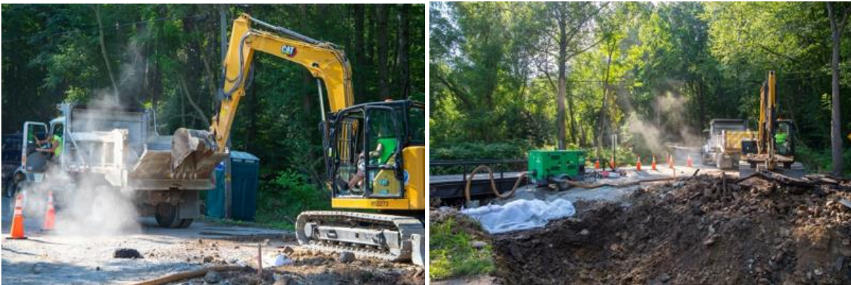
Swope Road Culvert Replacement project
