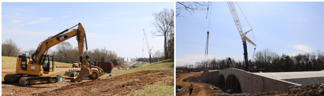
Halfway Boulevard Extension project
